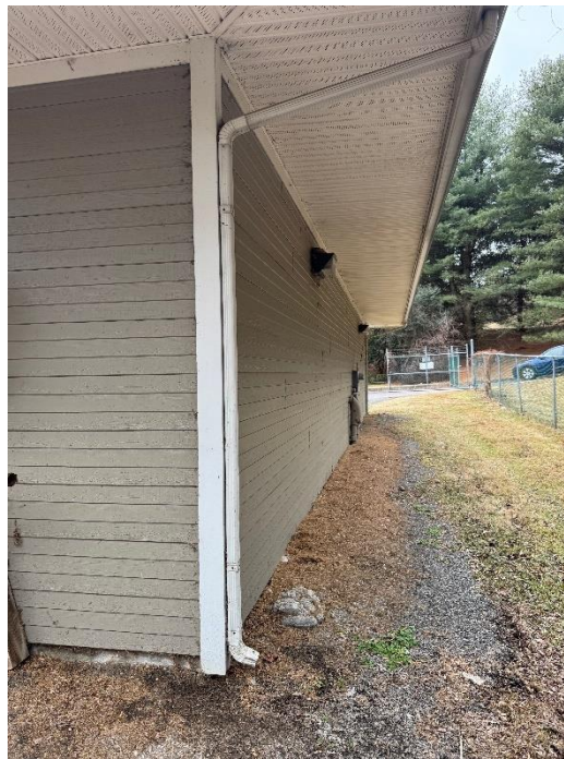
Photo No. 10: Western Side of Control Building
