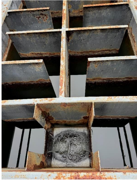
Photo No. 5: Existing Chlorine Contact Tank
