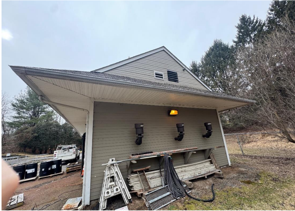
Photo No. 9: Northern Side of Control Building
