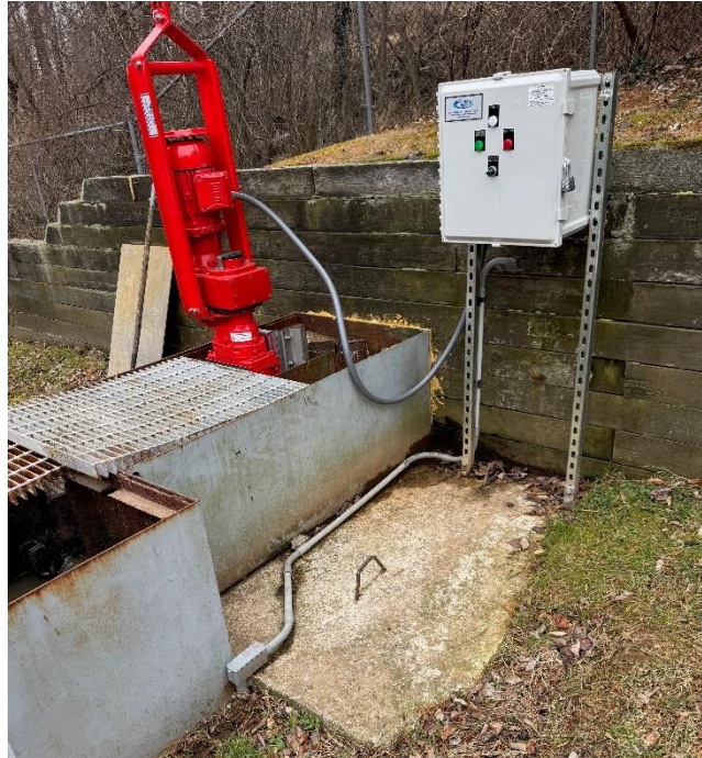
Photo No. 1: Existing Headworks (Sewage Grinder)
