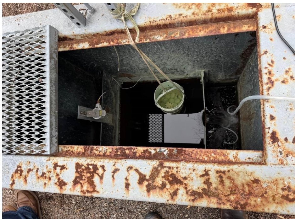
Photo No. 4: Existing "Dechlorination Tank"
